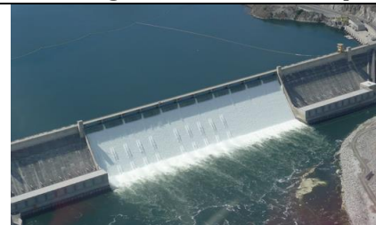
Energy generated by Grand Coulee daily.
